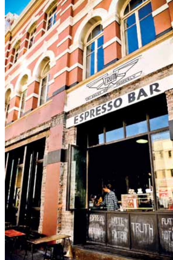
A Central City with a vibrant mix. The contemporary exterior of the CTICC in the financial district of the Foreshore complements heritage buildings (left) in The Fringe .
